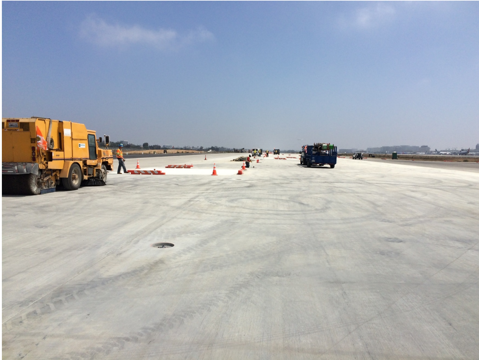
Runway 24R pavement and centerline lights - 8/24/15
