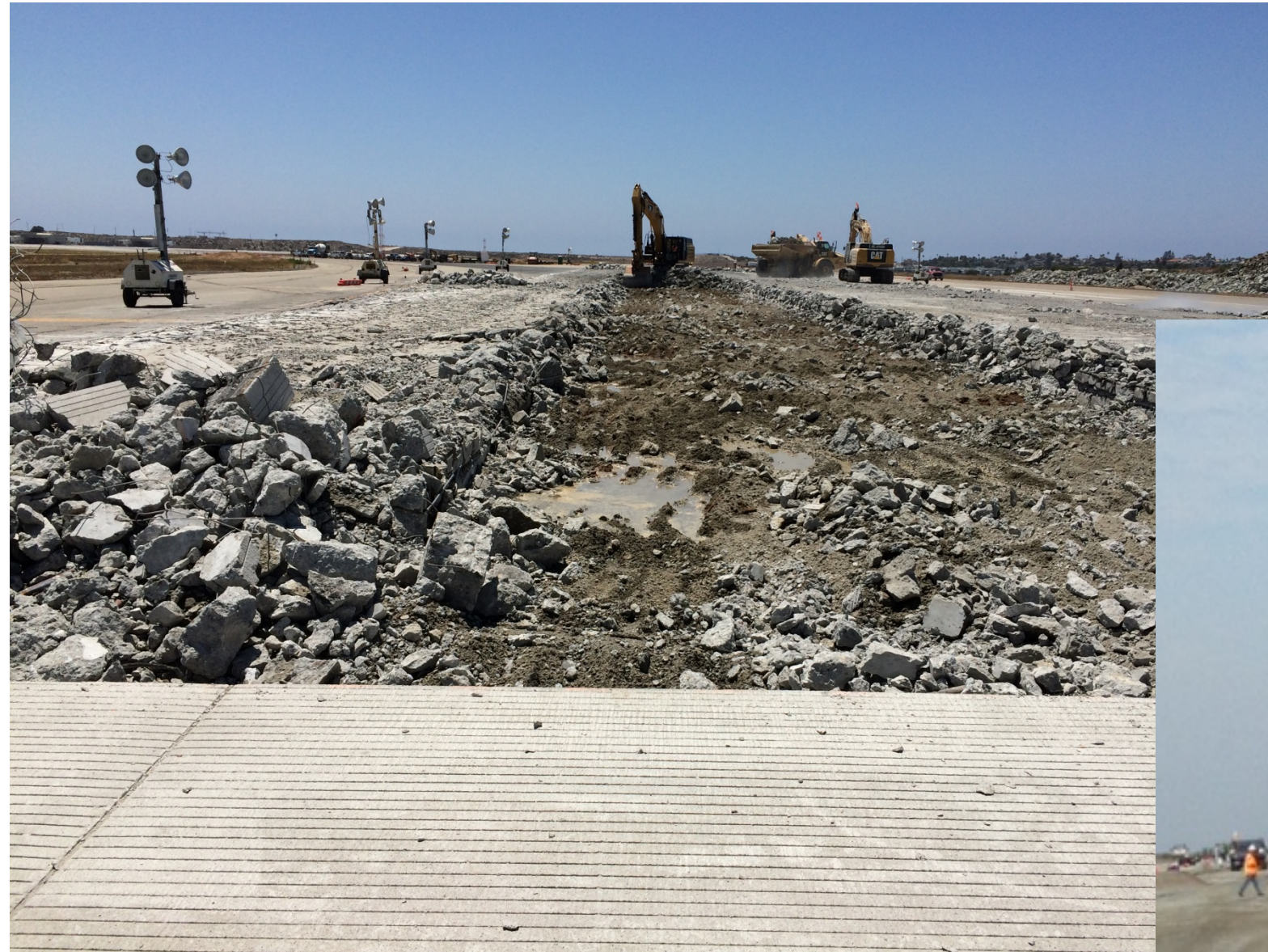
Runway 24R demolition - 7/13/15
