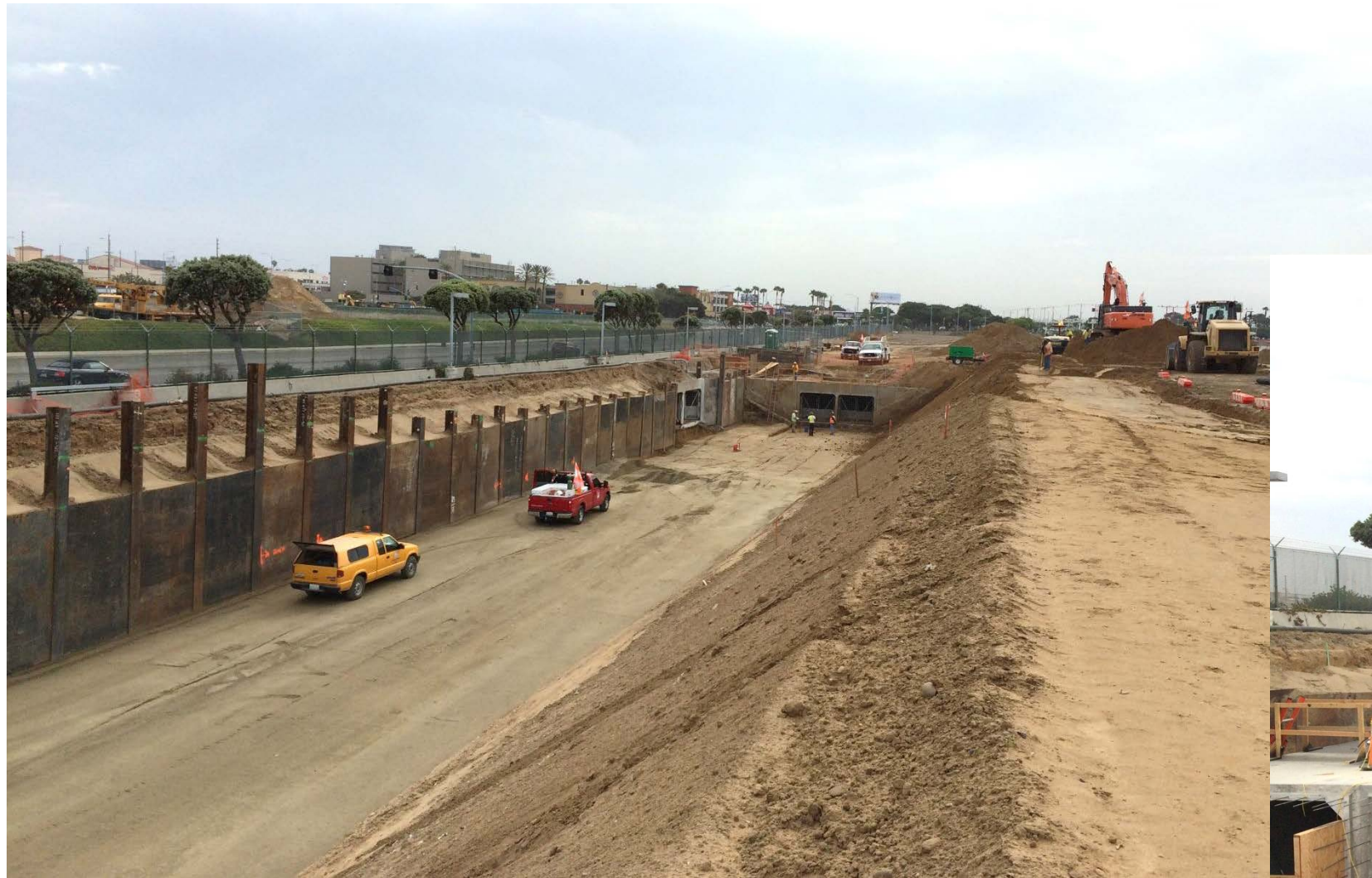
Argo Channel shoring and grading – 7/30/15
