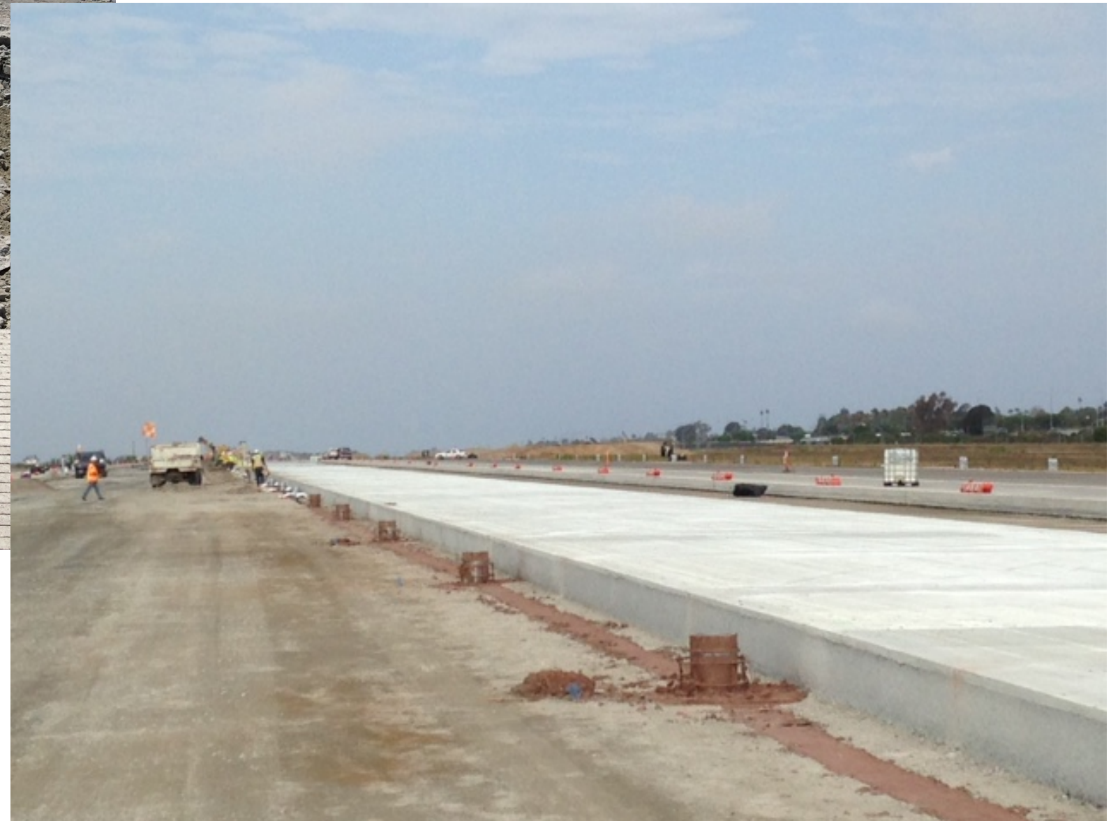
Runway 24R paving lane and centerline light cans - 7/29/15
