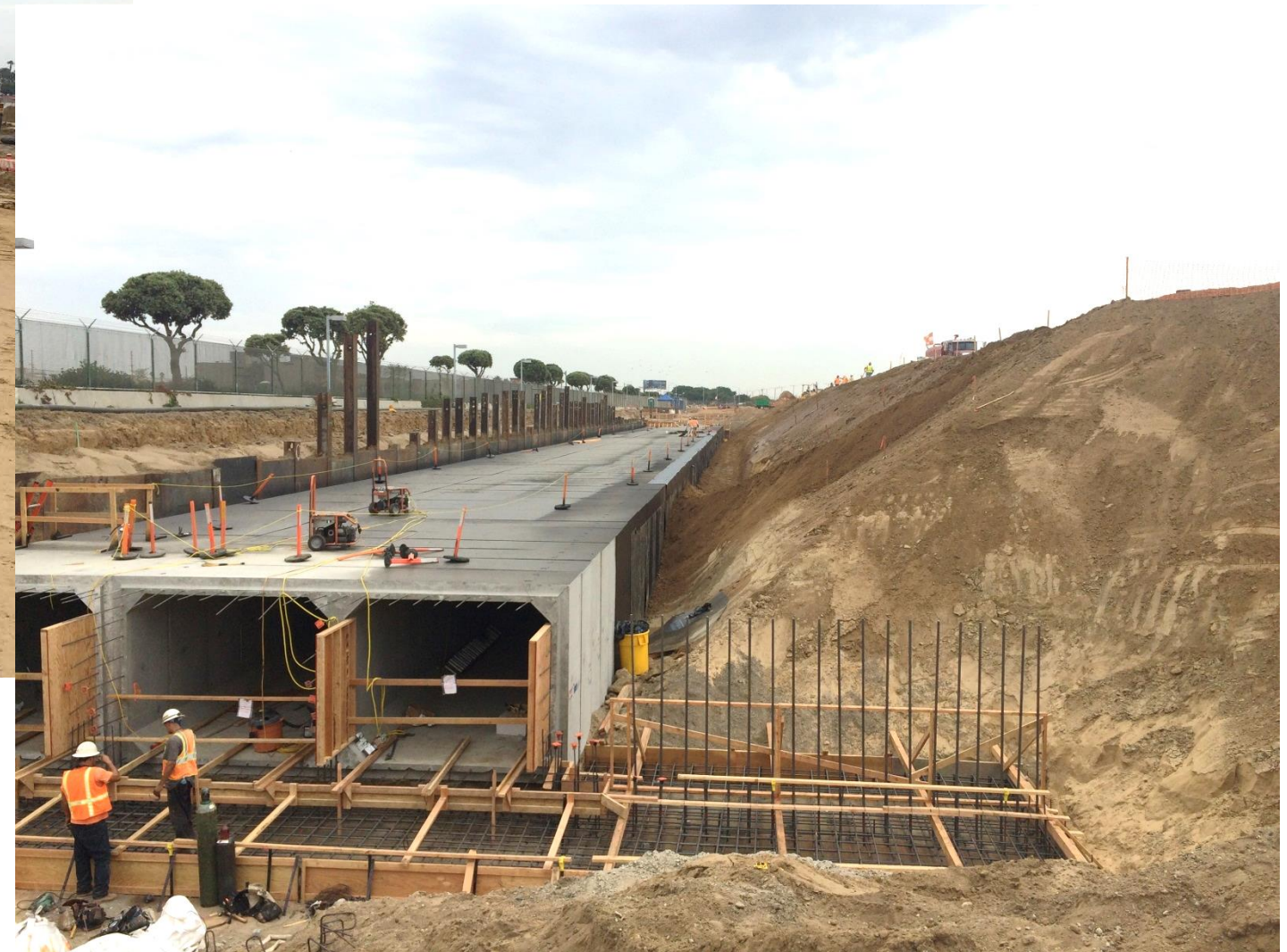
New Argo Channel box structure – 8/25/15
