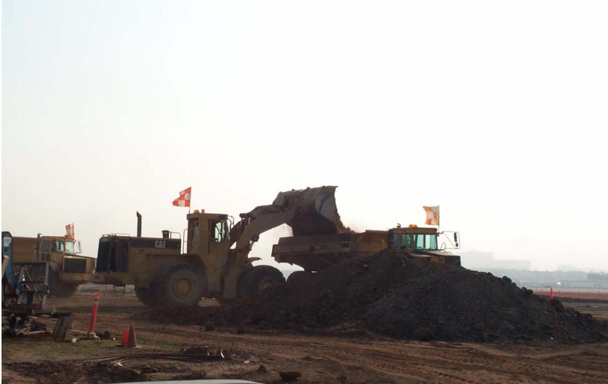
*Figure 6.-7 Excessive Dust Emissions Created During Loading Operations*
