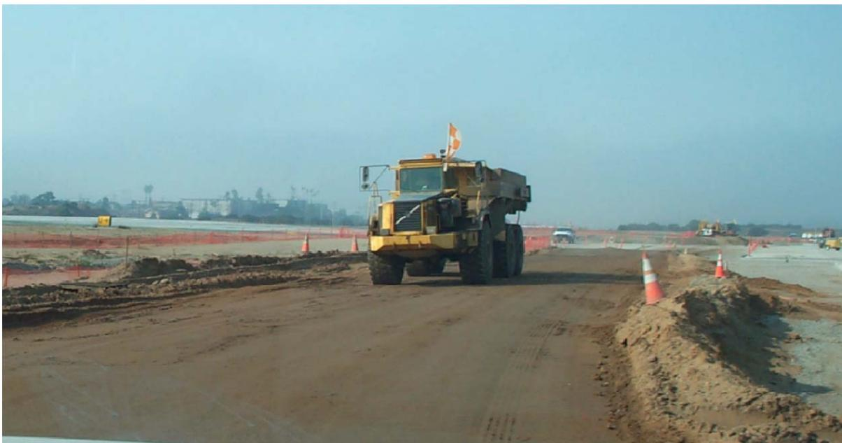
*Figure 6-6: Haul Roads are Kept Wet to Reduce Fugitive Dust Emissions*
