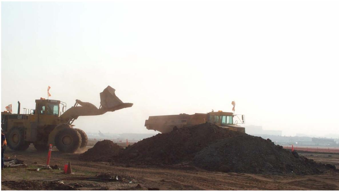
*Figure 6.-8 Excessive Dust Emissions Created During Loading Operations*
