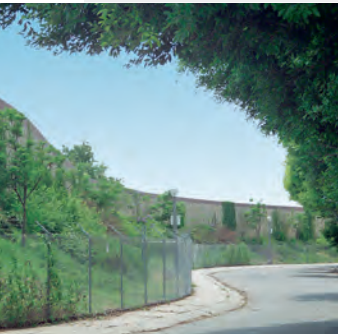
Landscaped earth berm and concrete sound barrier (above) help reduce the impact of aircraft noise in communities immediately surrounding LAX.
