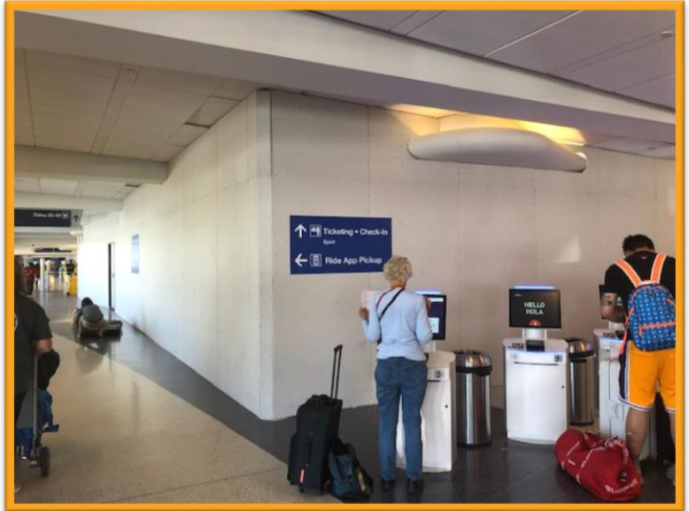
Terminal 5 Ticketing: Construction Barricades
