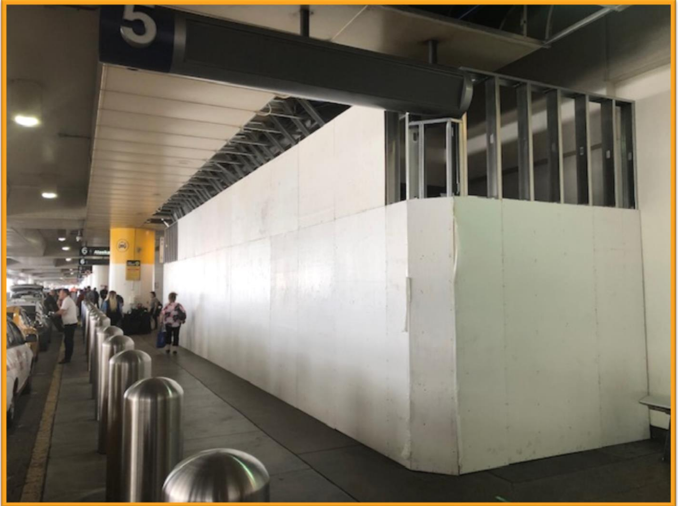
Terminal 5 Arrivals Level: Sidewalk Restrictions & Construction Barricades
