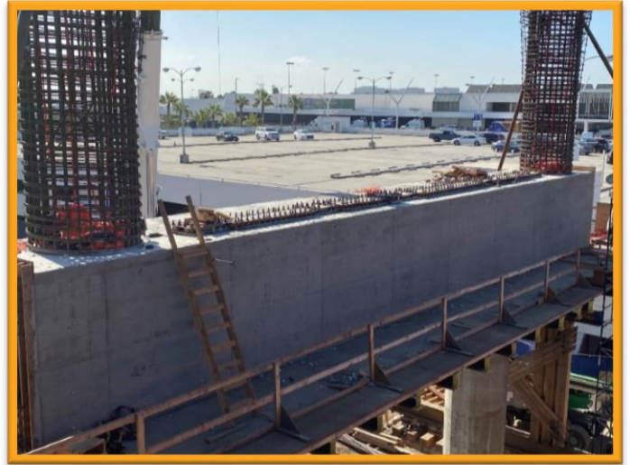
APM East Station as of Monday, May 4 (two weeks ago)
