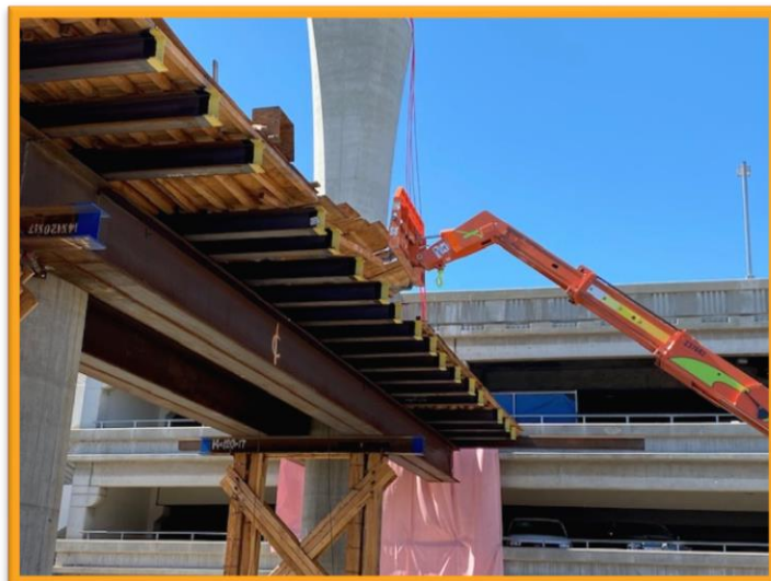
Above: Falsework is removed from an East CTA Station bent
