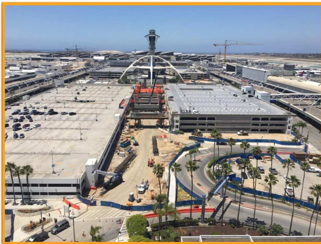
Above: Falsework is removed from an East CTA Station bent
