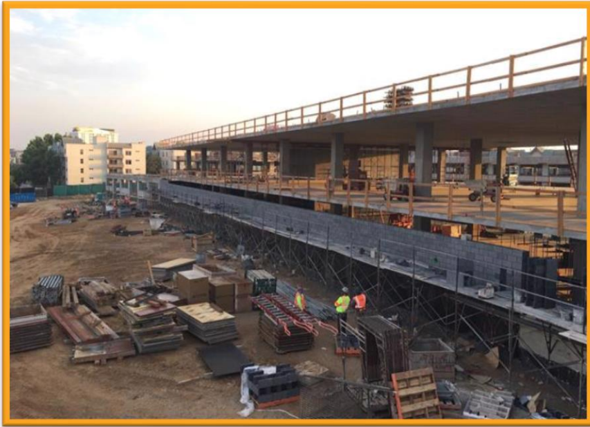
APF's final concrete pour on Parking Structure roof
