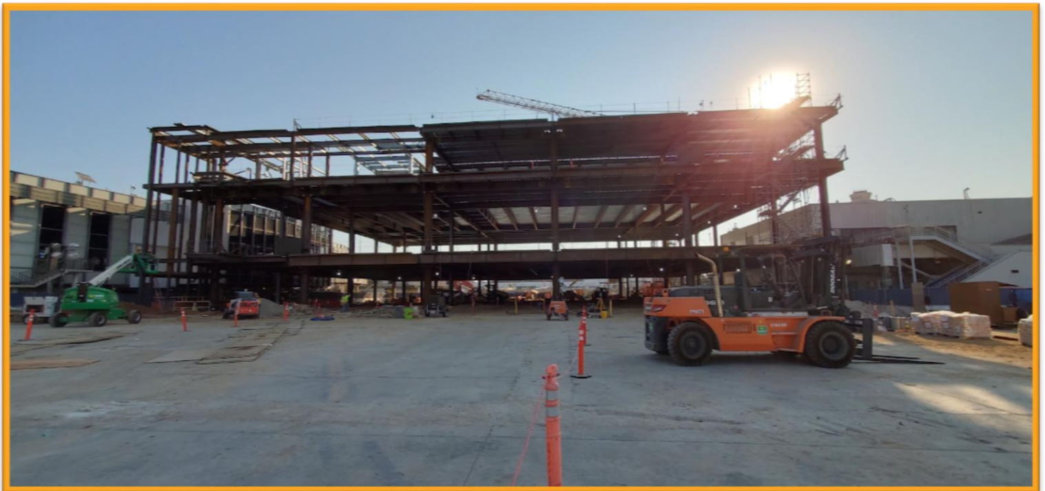
Terminal 3 Construction Progress
