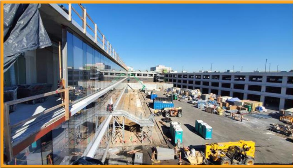
Ongoing construction of the Airport Police Facility and Parking Structure
