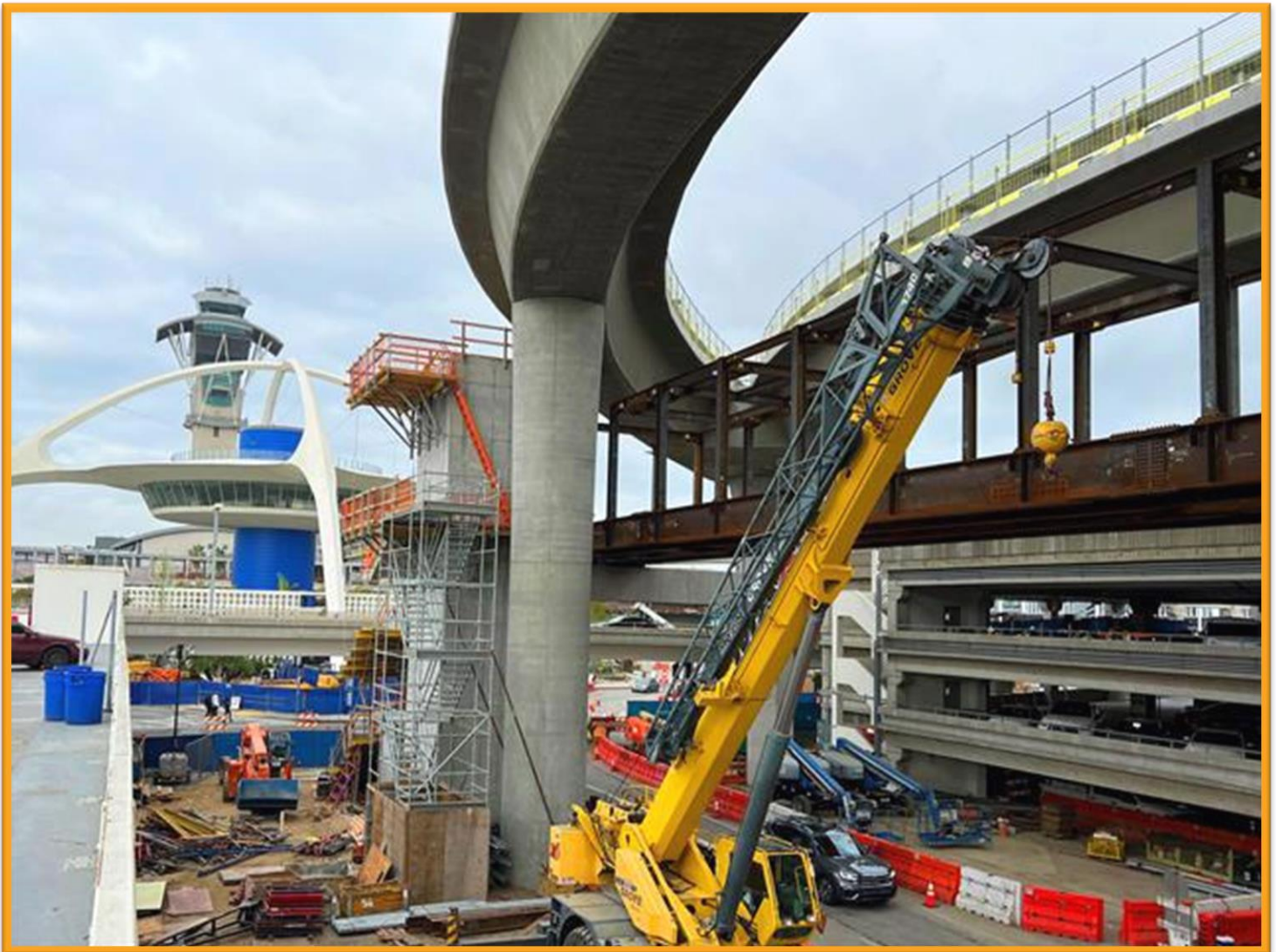
Crews work to set the final structural steel at the APM's East CTA Station, as part of the future Theme Building Viewing Pavilion
